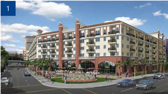
300 North Beaudry Avenue, Los Angeles, CA
