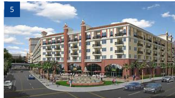
300 North Beaudry Avenue, Los Angeles, CA
